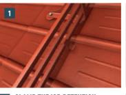
**CLAMP THE ICE-RETENTION** BRACKET ONTO THE PIPE
