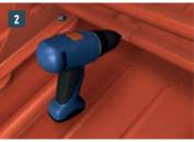
2 FASTEN THE ICE-RETENTION **BRACKET USING THE FASTENING SCREW SUPPLIED WITH** THE BRACKET
