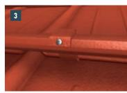
3 FULLY INSTALLED **ICE-RETENTION BRACKET**
